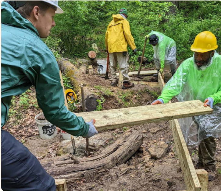
LandForce Pittsburgh, trail structures and carpentry training
